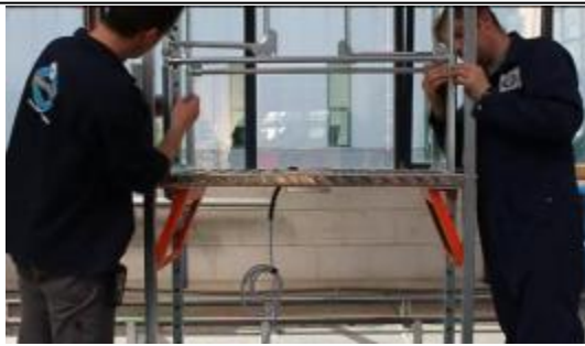
Fit the bars of the rail
