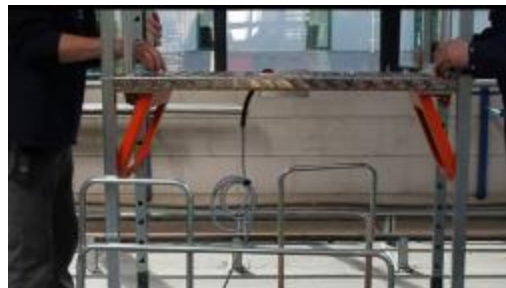
fit the poles for the rail
