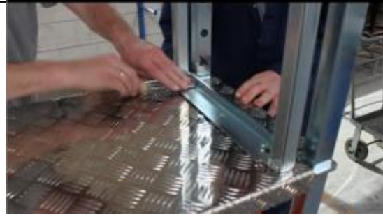
secure the rail with the bolts
