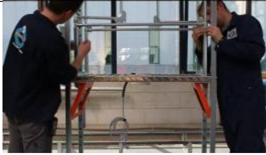
Fit the bars of the rail
