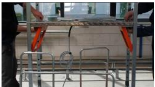
Remove the bolts for the rail
