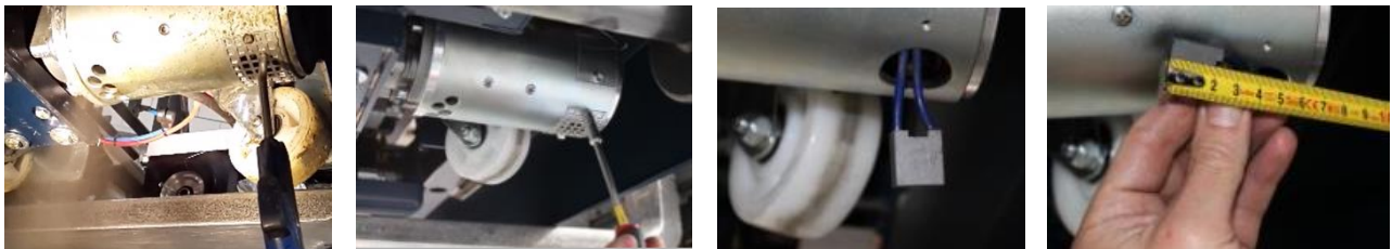
Figure 9.4; Inspecting carbon brushes in the motor
