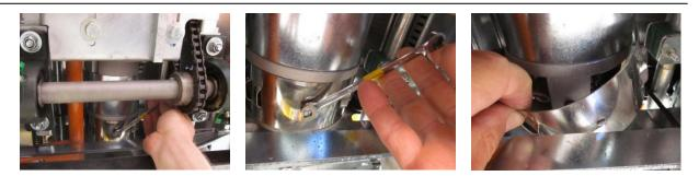
Remove the brush cover with 8mm spanner.
